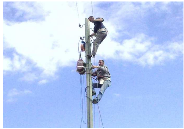
Mounting VROT-18-1 onto the pole
