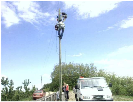
Lifting VROT-18-1 onto the pole
