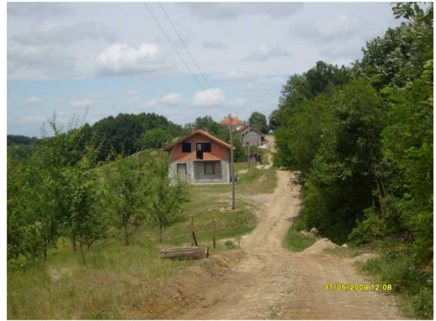
Rural municipality area supplied energy through VROT-18-1
