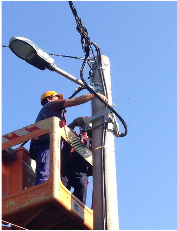
Installing console for VROT-18-3
