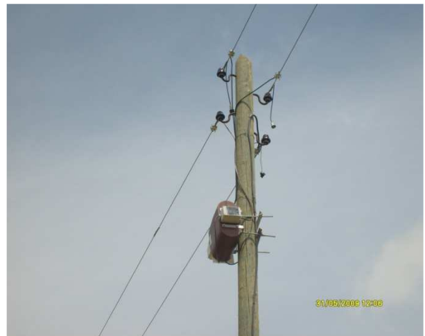
Lightning overvoltage destroyed surge arrester and VROT-18-1 not damaged at all
