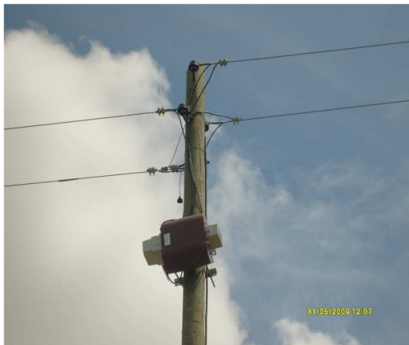
VROT-18-1 mounted on the pole
